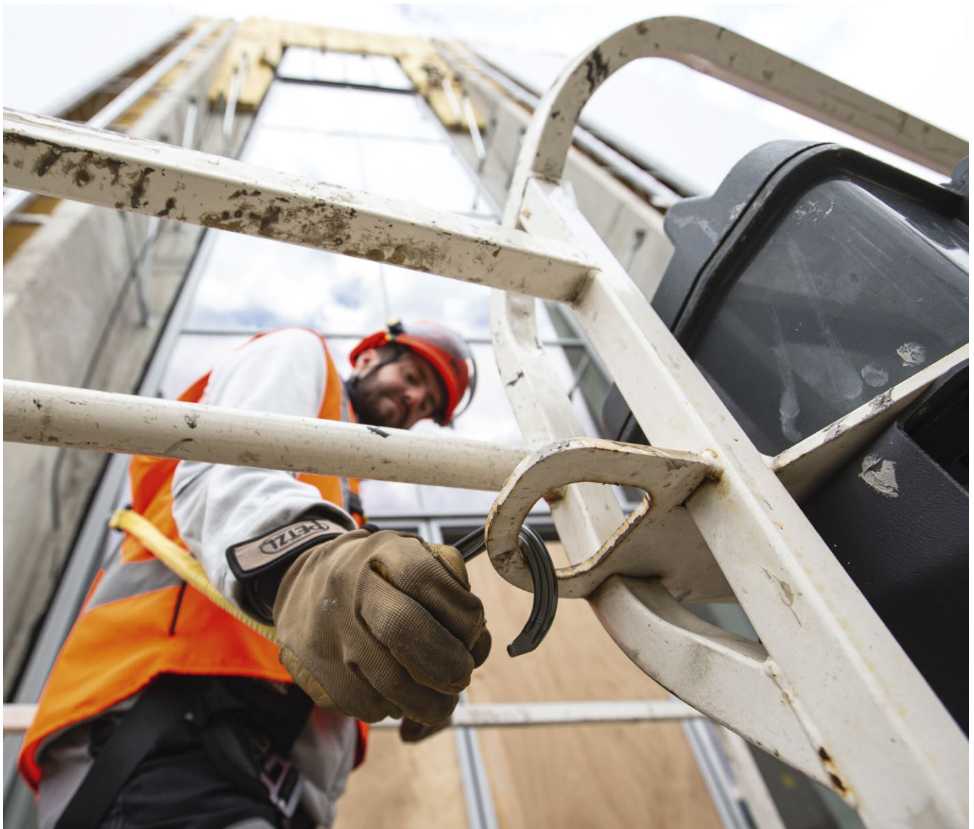
Glass window construction at the new Petzl testing facility, Crolles, France. © Petzl Distribution - Latouche
